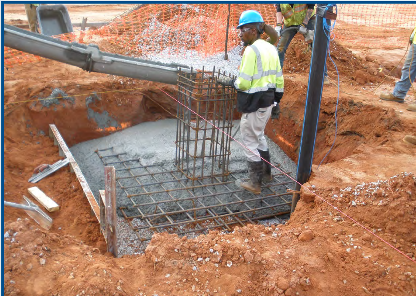
Concrete column pouring, September 2023.
