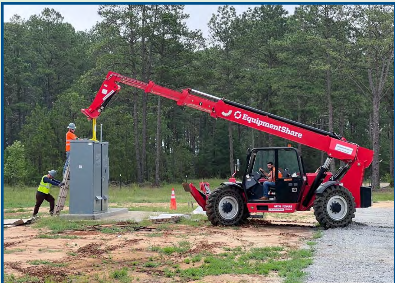
A Motor Control Center being installed, July 2024.
