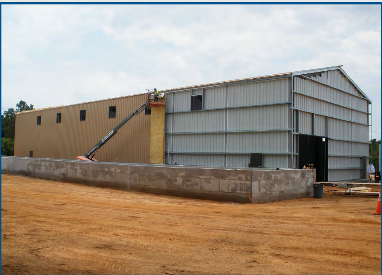
Insulation/siding being installed on the Pre-Engineered Metal Building, June 2024.
