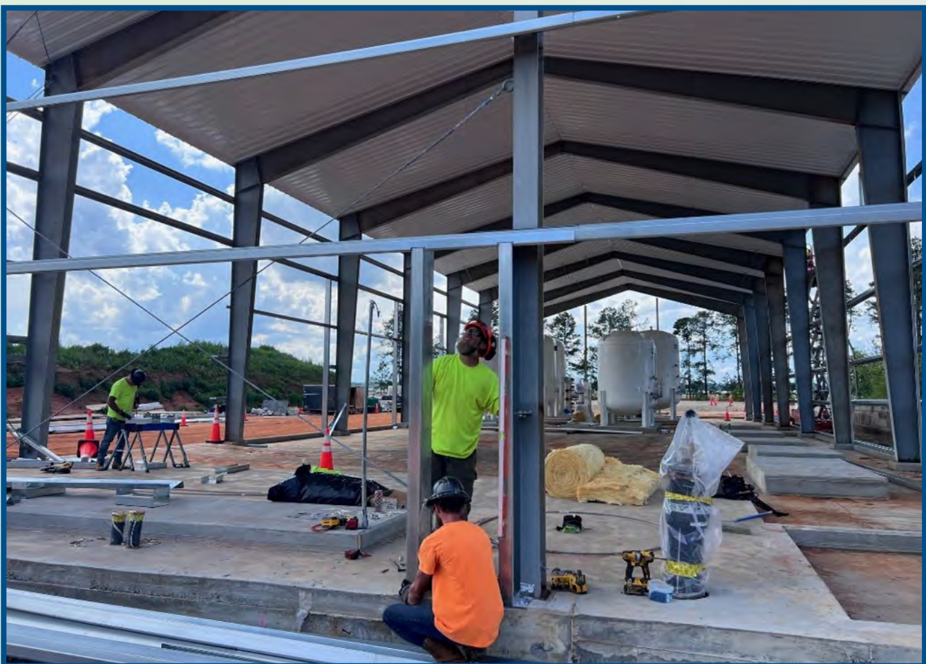
Installation of Pre-Engineered Metal Building Girts and Framing, May 2024.
