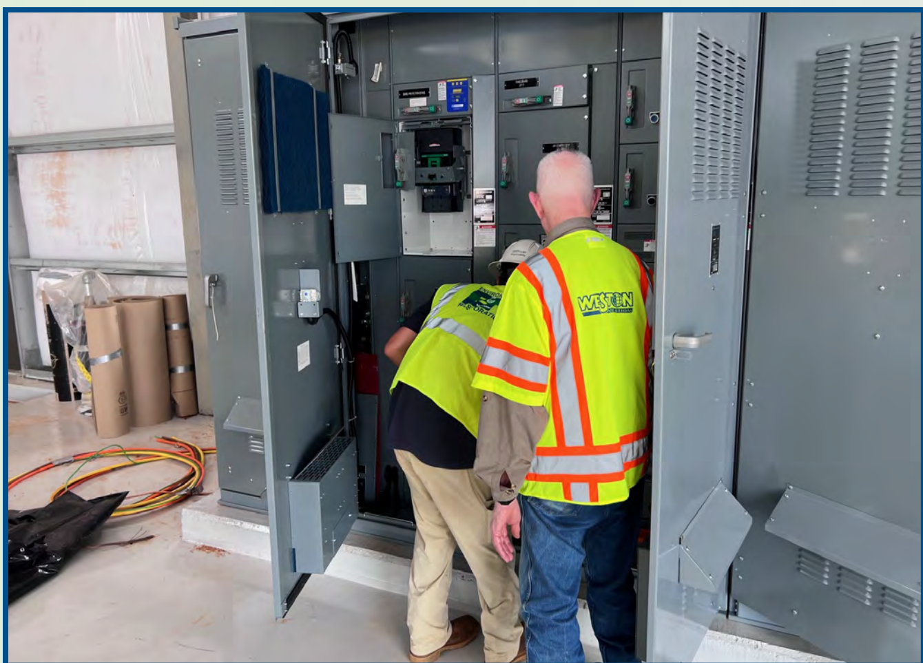
Inspecting breakers in the Motor Control Center, July 29 2024
