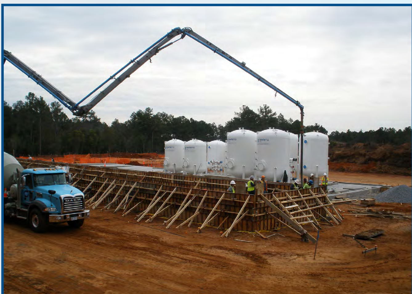
Pouring concrete into Tank Farm concrete wall forms, February 2024.
