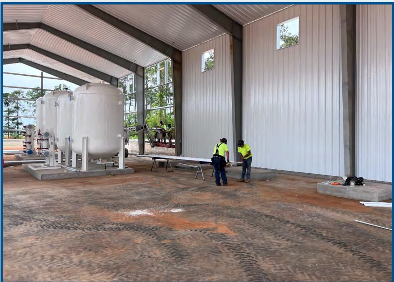
Interior liner panels being cut to fit in the interior of the Pre-Engineered Metal Building, June 2024.
