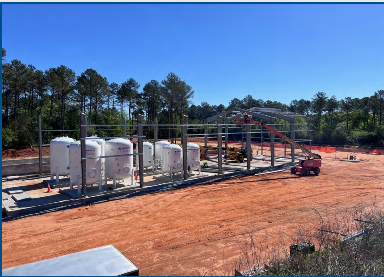
Erection of the Pre-Engineered Metal Building, March 2024.
