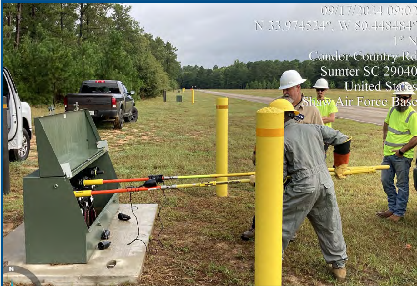
Sectionalizing Cabinet Work
