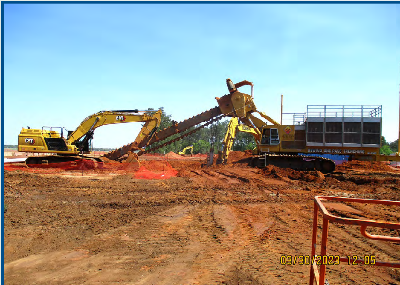
The 40-foot trenching machine, March 2023.
