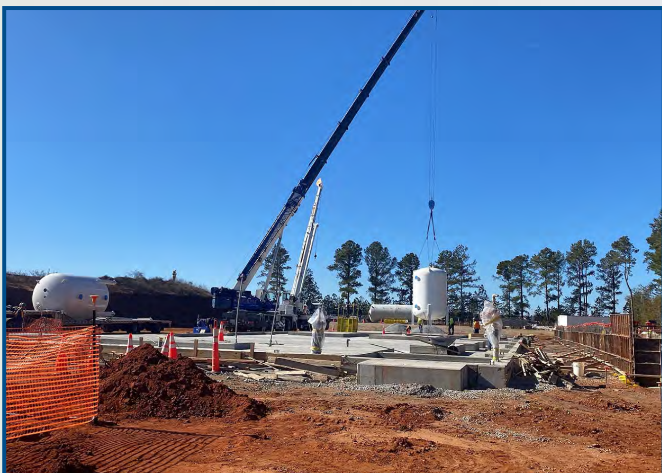
Installation of Ion Exchange Resin and GAC tanks, February 2024.
