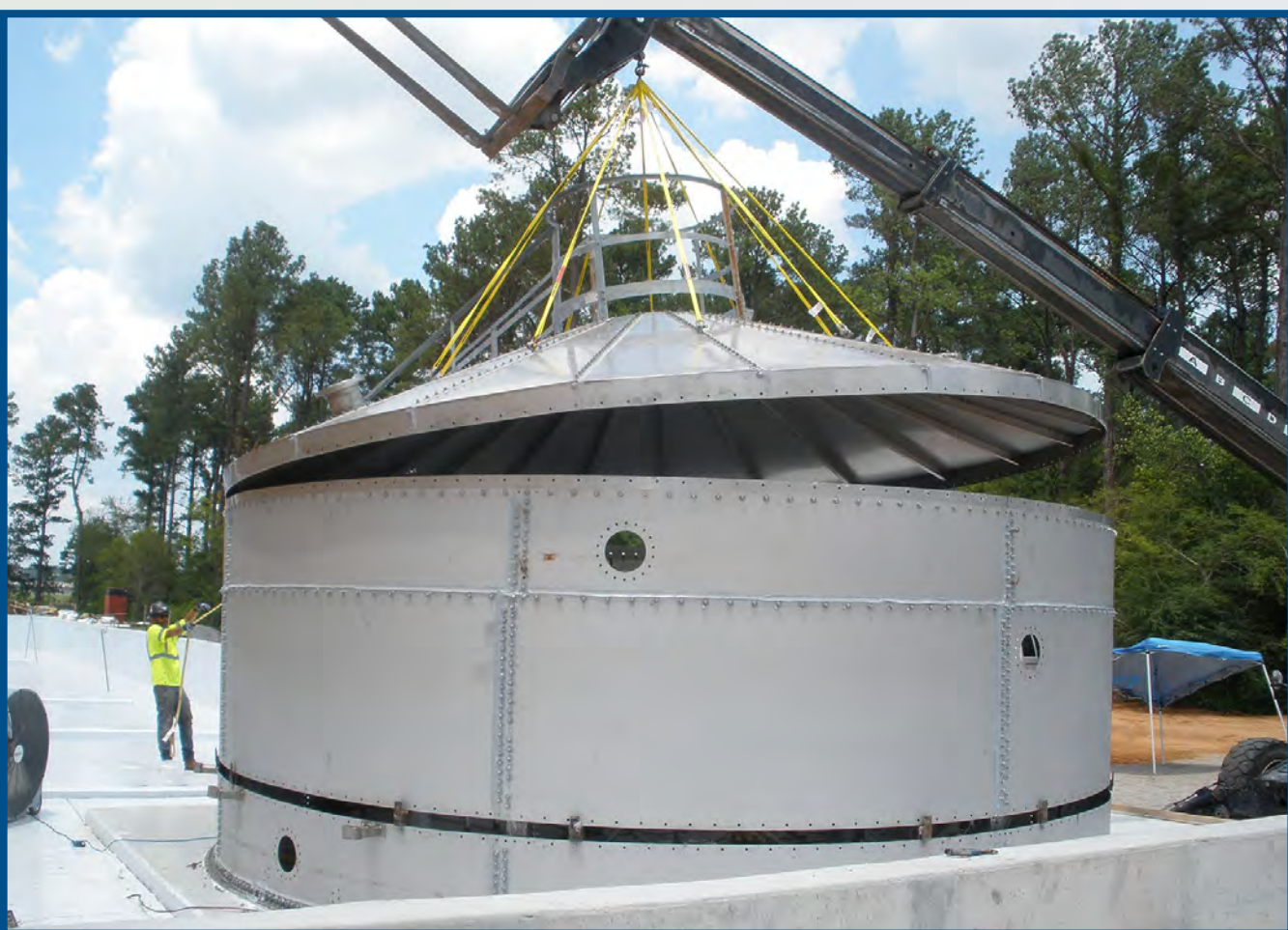
The top of the Field Erected Tank being installed, July 2024.
