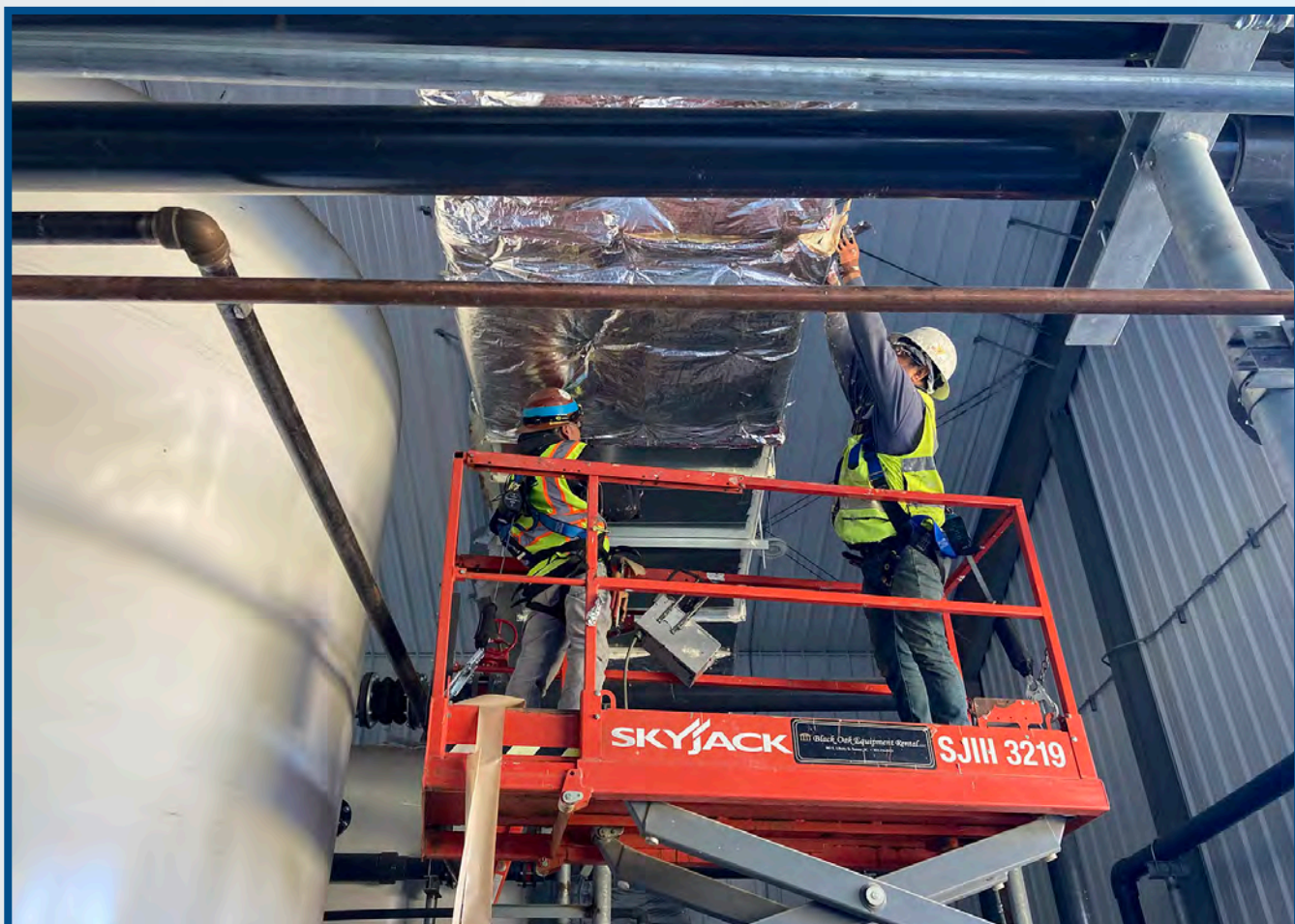
Air Duct Insulation
