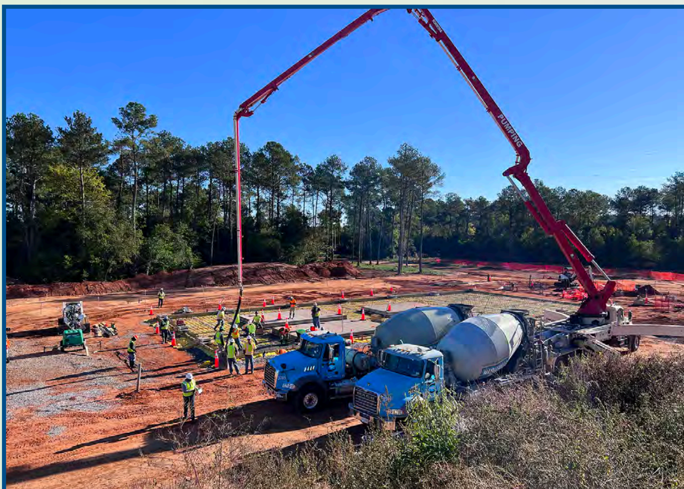
Groundwater Treatment Plant concrete floor pour, October 2023.
