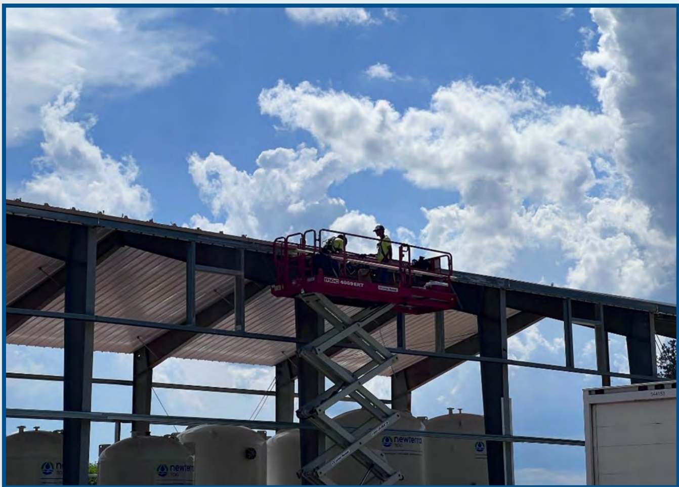
Installation of the Pre-Engineered Metal Building Roof, April 2024.
