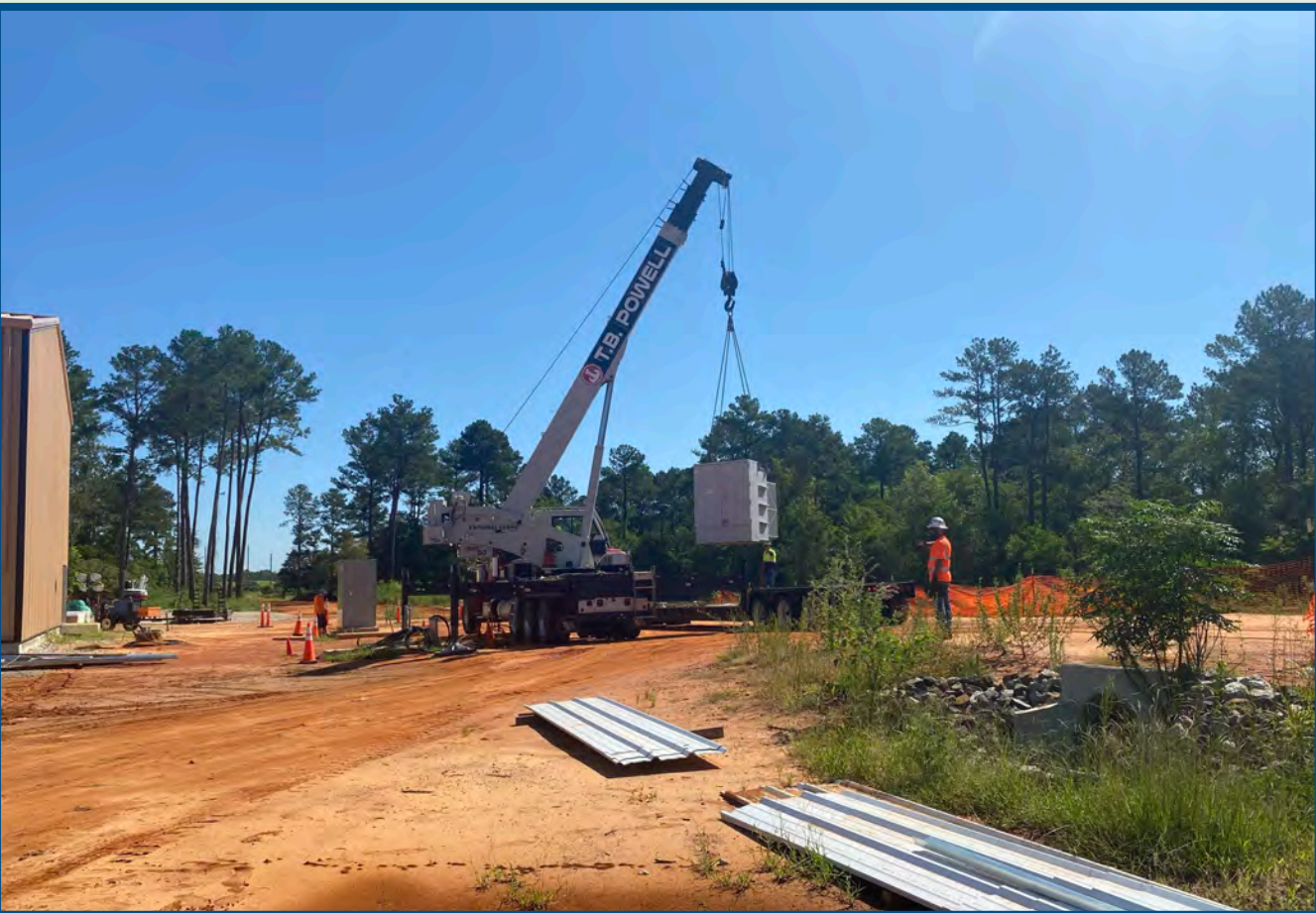
Transformer Installation
